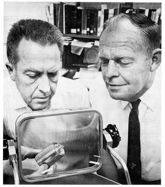
ASSEMBLED INERTIAL SWITCH is inspected by Larry Estabrook (2324), left, and E. R. Wood (4221-2). The device represents three months' work by the Development Shops to design and fabricate tooling and fixtures for assembly of the switch.
